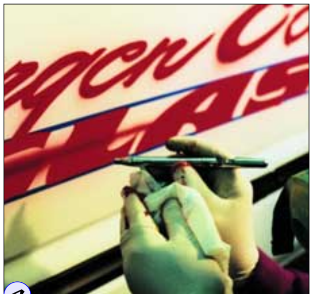
4 Now I mix up some maroon with the High-temp reducer (about 60% reducer to 40% paint) and apply my highlights, using my Iwata Eclipse airbrush at 45 psi. Notice that I'm using latex gloves for protection.
